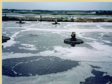
Basin Mixing and Air Distribution (Note: surface aerators are not in use)
