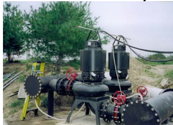
Dry Sump Centrifugal Pumps
